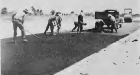
SOUTH of the Palm Beach Club workers level out asphalt and crushed stone to be packed smooth by the roller in the background. PA ZUID of Palm Beach Club tradadonan ta plama asfalt y pedra granu canal to worde pisa door di e roller patras.
